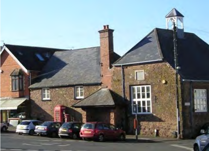
Figure 44 (above): Former Boys School, The Square
