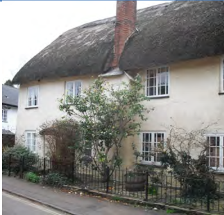
Figure 12 (above): 28 Fore Street
