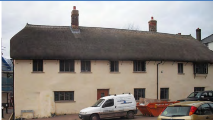
Figure 30 (above): 1 Fore Street
