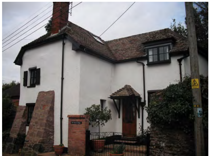
Figure 28 (above) 2 Tiverton Road
